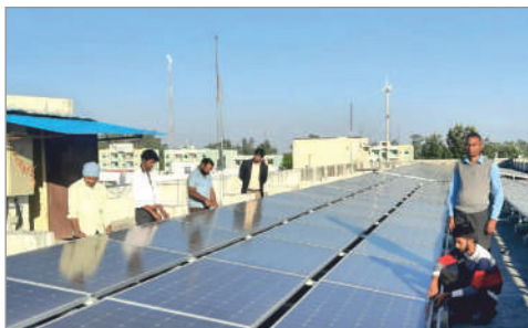
Installation of 150 KW Roof top solar plant by CRE Bhopal RNTU
